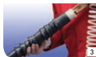
3 Begin to remove the inner core, allowing the termination to shrink down onto the cable
