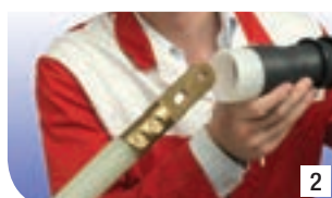
2 Place the 3M™ Cold Shrink Termination Body over the cable end and position at the correct point on the cable
