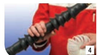
4 Once the inner core has been fully removed, the termination installation is complete!
