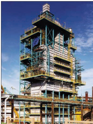
Ethylene Cracker Unit
