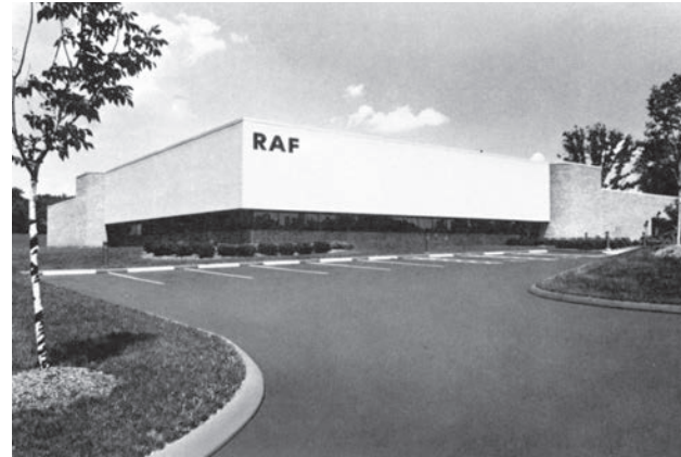
U.S. manufacturing and plating facility
